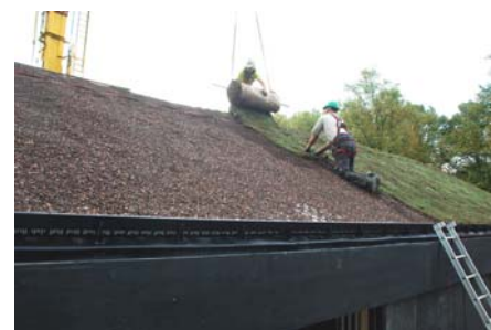
After leveling the substrate layer, the vegetation mats were applied.
