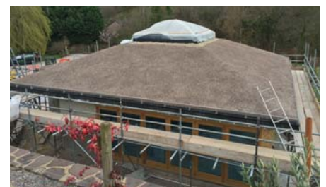
Before applying the sedum plant mats the system substrate was leveled.
