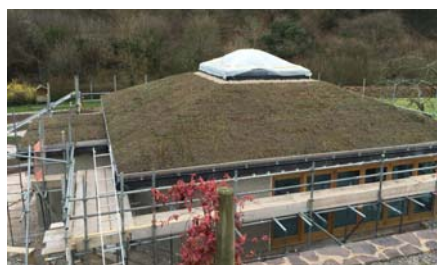
The sedum mats were laid close together, without overlapping.
