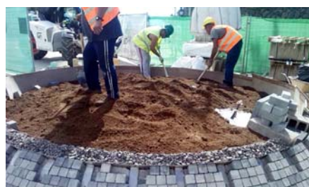
The drainage elements were covered with 100 mm of system substrate.
