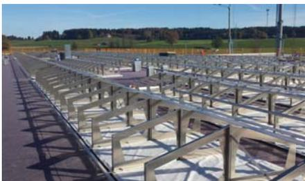
The Solar Bases SB 200 were first covered with a filter sheet, then the Solar Base Frames SGR were attached.
