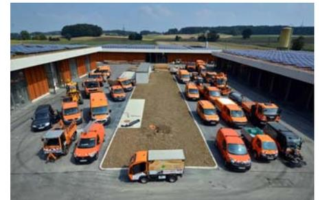
On the roof of the left building the solar panels were installed with an east-west alignment, on the other two buildings, the "classic" orientation to the south was chosen.
