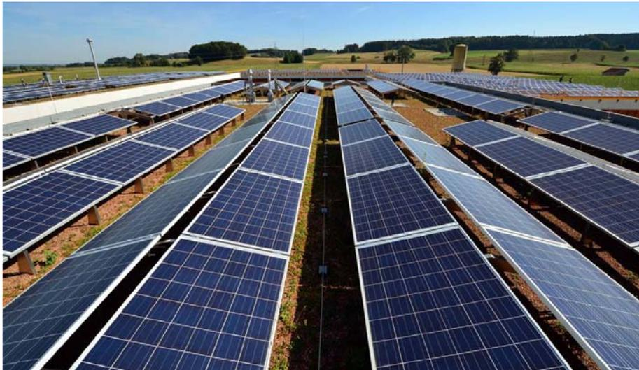
In order to have a uniform energy yield throughout the day, one part of the solar panels was oriented to the south, the other part, which is visible on the picture, was installed with an east-west alignment.
