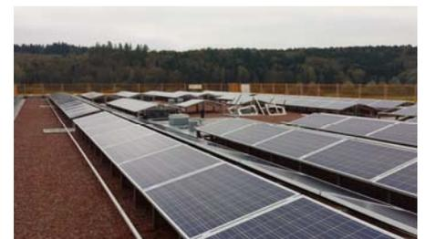
A rail system for fall protection was attached additionally to the Solar Base SB 200.
