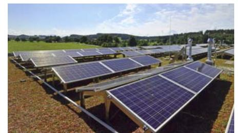
One year after completion a slight green coverage is visible. The photovoltaic system covers not only the consumption of the buildings themselves, but also supplies nearly 100 households with "green electricity".
