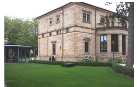
Fixodrive® FX 50 was applied even under the lawn area.
