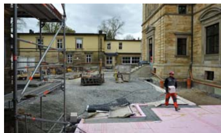
On top of the inverted insulation the extremely stable, air and vapor permeable Filter Sheet PV is first installed. Then the Fixodrive® FX 50 with an attached filter sheet is rolled out. A gravel layer provides a base for the paving and its bedding.
