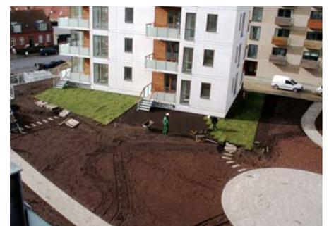
After completion of the rough works on the underground garage roof, the turf in the private gardens was laid.
