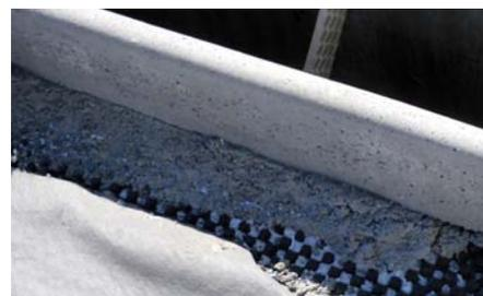
Floradrain® FD 25-E is used as permanent form-work for the separation between hard surface and garden.
