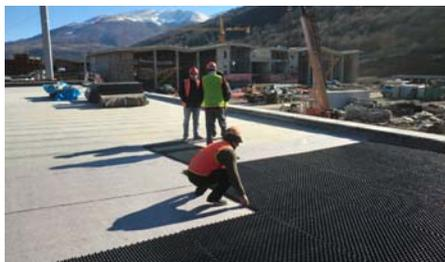
The drainage elements were laid butt jointed on all roof surfaces.
